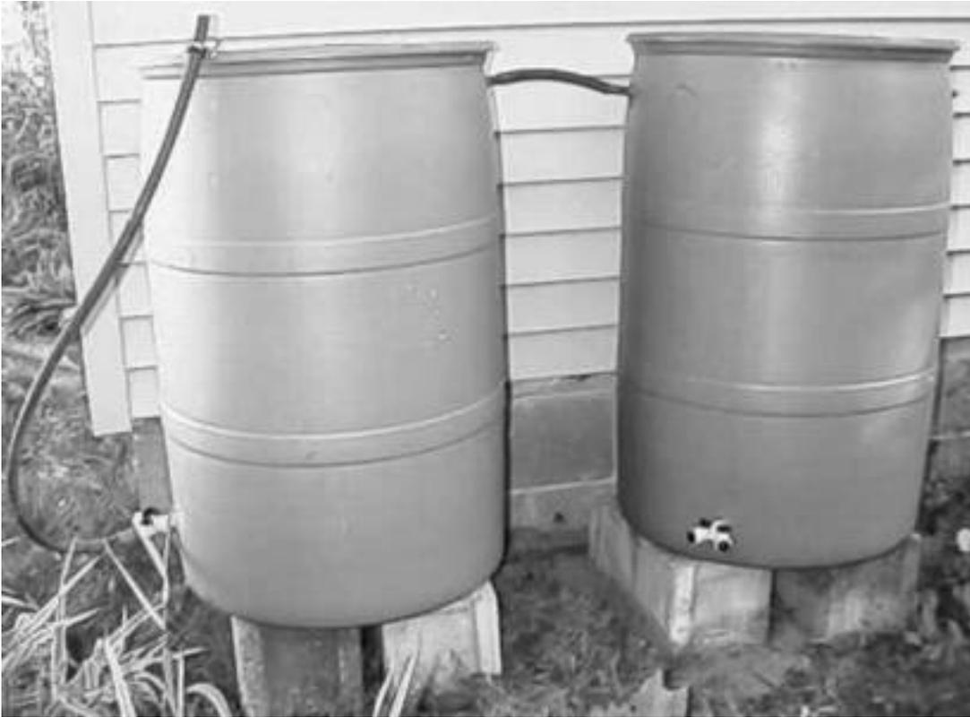
In the above photo, note the short hose connecting the two barrels. This is the overflow line. When the first barrel becomes full, additional water will simply flow through this hose into the second barrel. When the second barrel becomes full, that overflow hose will drain onto the ground away from the foundation.
